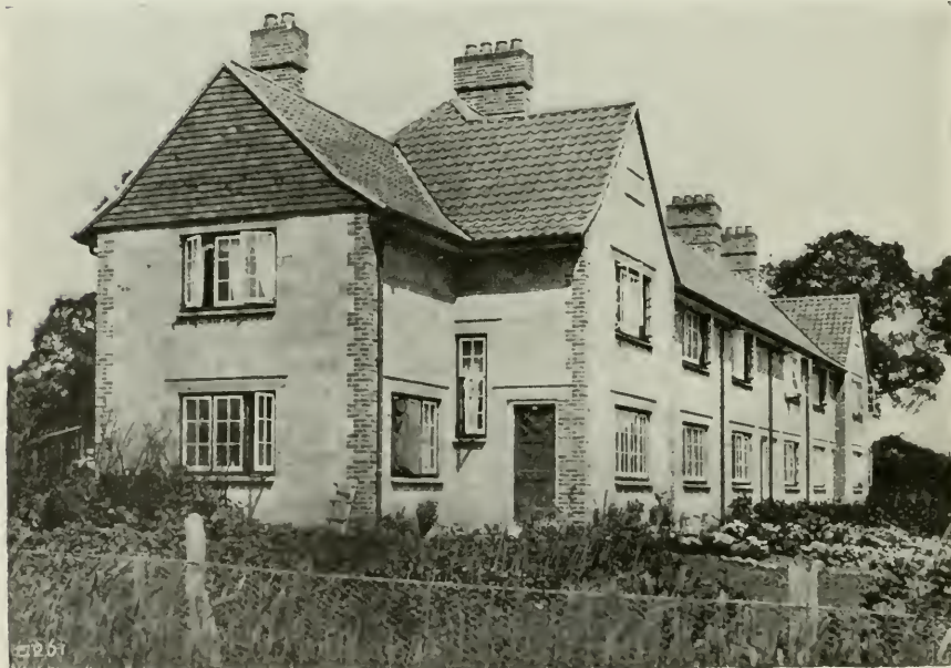
FIGS. 28 AND 29.—CONCRETE COTTAGES, WHITLINGHAM, NORWICH.
